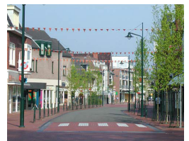
A raised and paved intersection extends the language of the sidewalk to the street.
