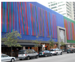
16 Integrated Facade System Fifth Third Bank Center Garage Julian Stanczak Cincinnati, OH, United States
